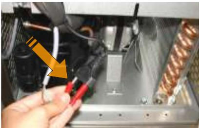
**4.** Connect the agitator pump terminal at back of the cooler.
